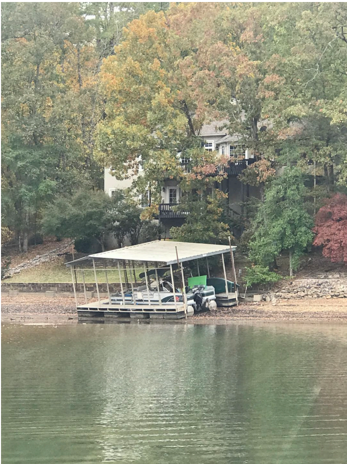
Figure 5: Dock and boat resting on the bottom after the drawdown
