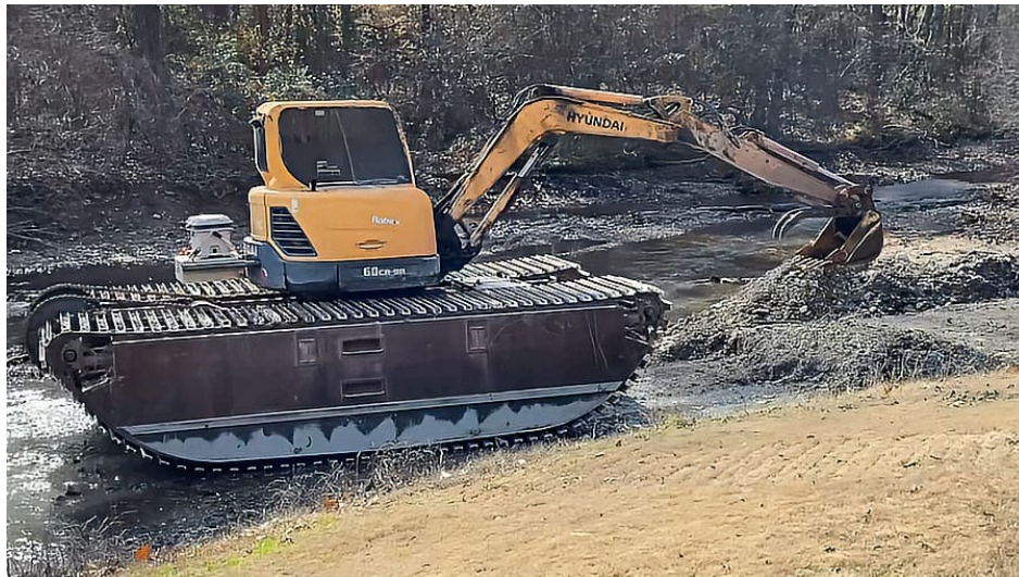
Figure 3: Amphibious dredging machine working on silt removal on Cortez Lake
